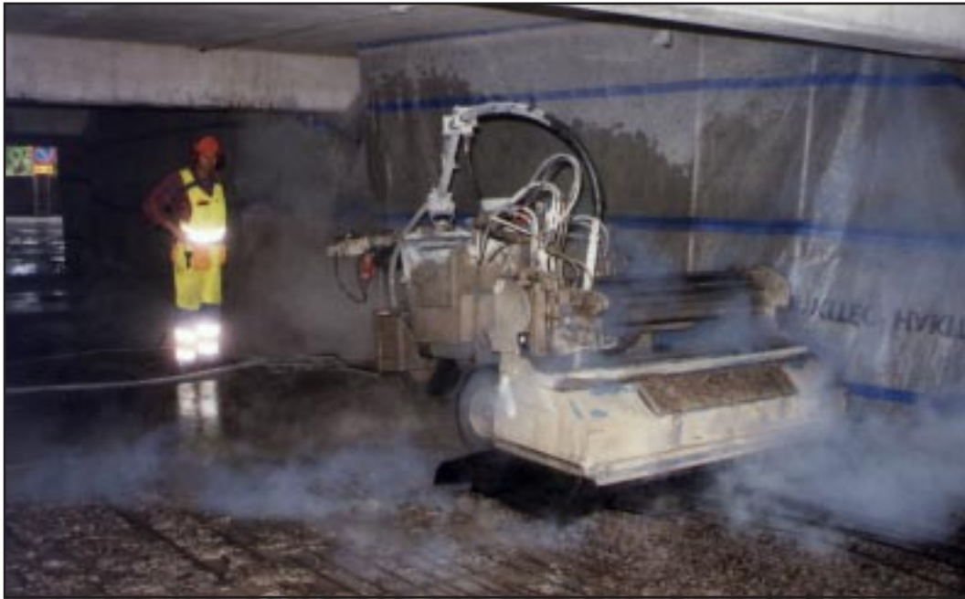
The Conjet Robot 230 at work in the carpark.
