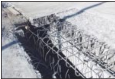
Edge beam rebars exposed by hydrodemolition
