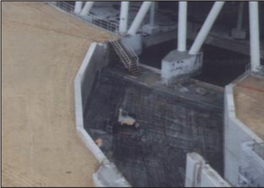
The Conjet Robot is working on the cooling water feed channel.
