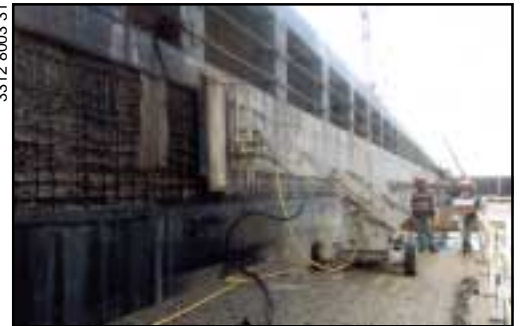
Strips of damaged concrete was removed from the dock walls.
