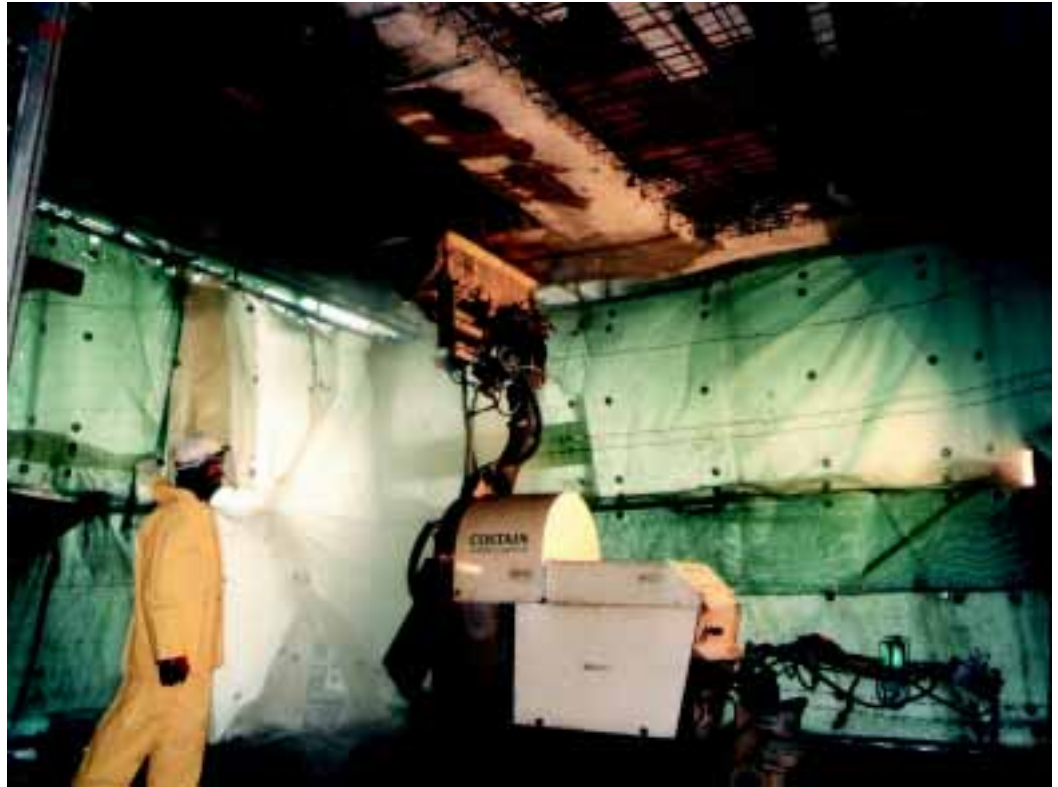
Conjet Robot 360 equipped with boom extension arm.
