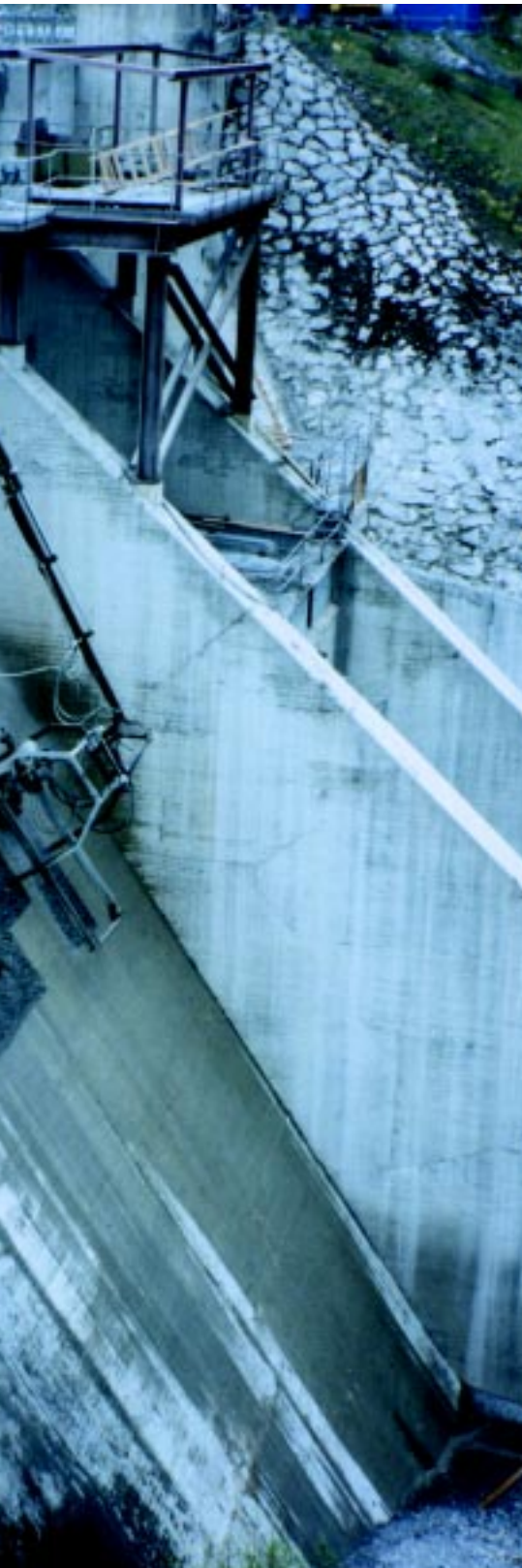
Surface at the water intake hydrodemolished down to the rebars by a Jetframe from Conjet.
