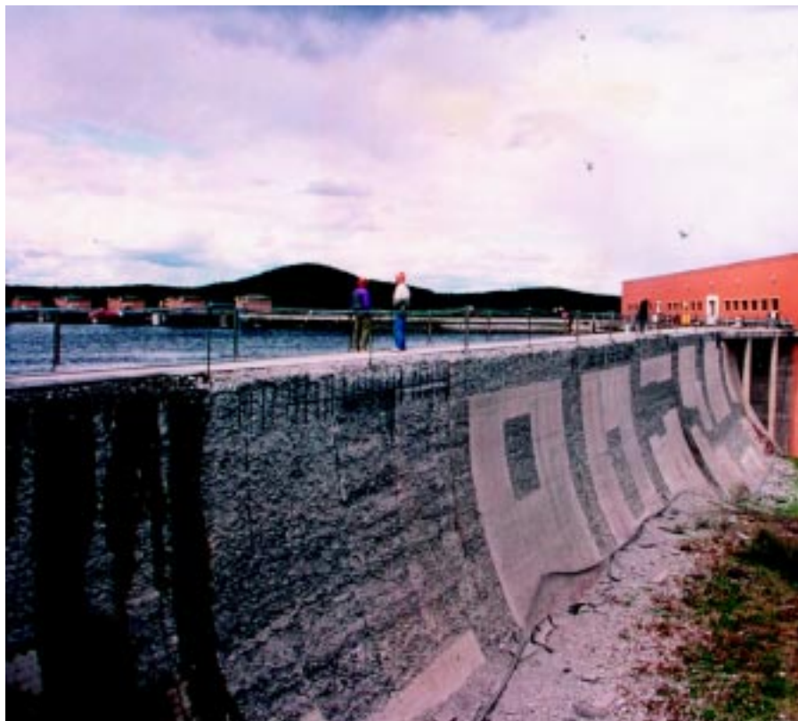
Surface at the water intake hydrodemolished down to the rebars by a Jetframe from Conjet.
