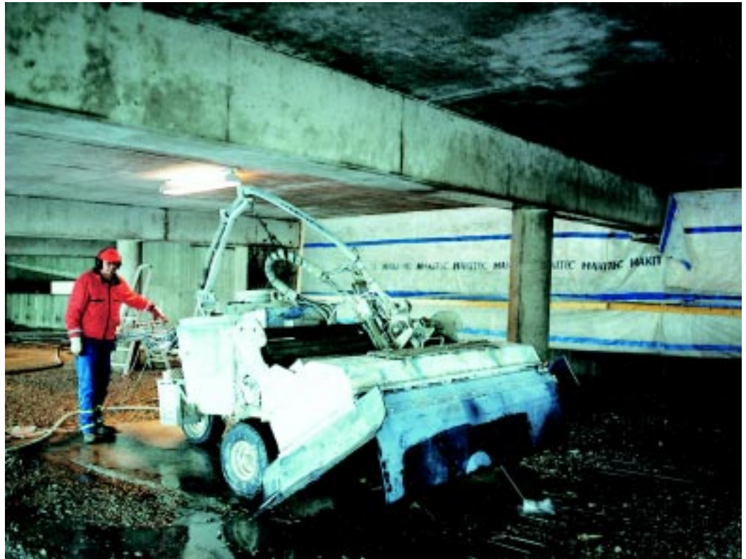
The Conjet Robot 230 at work in the carpark.
